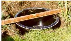
Lift off the first hole for the basin. Enter all around the excavation to about 5 cm so that you can easily align the basin. Then, align the basin using a spirit level accurately. Filling the remaining voids with earth again.
