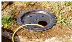
Fill the basin with water. Check again that the basin is well slurred and can no longer be moved. Put on the lid and place the large opening in an easily accessible place.
