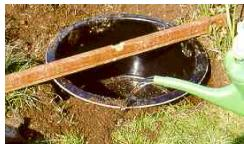
Sludge the basin with water. Check several times by means of a spirit level, the correct position of the basin.
