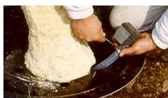
Place the water feature on the cover and run the hose connection back into the hole of the lid into the bowl (the large opening for the pump). Now connect the pump and insert it into the pool filled with water.
